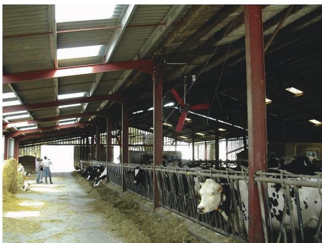
The **DAIRY FAN** is based on the biggest fan in the program of Vostermans Ventilation (the Multifan 130), with a size of 130 cm, which results in a very high air volume: 48.500 m<sup>3</sup>/h at 0 Pa. The dairy fan combines a high throw of 146 m and a high efficiency (26,2 Watt/1.000 m<sup>3</sup>/h).
